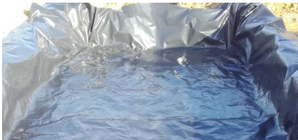
Figure 23 – Installation de la membrane souple
